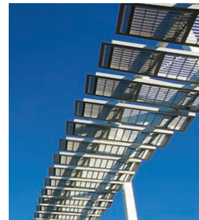
Solar panels at Whitehall Ferry Terminal.
